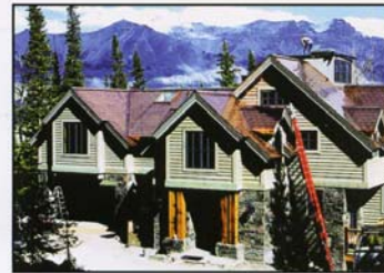
Known for its beauty, ease-of-installation, long lifespan and high performance in extreme weather conditions, copper shingles are becoming a popular roofing material, especially among high-end homeowners. Photo Courtesy of Revere Copper Products
